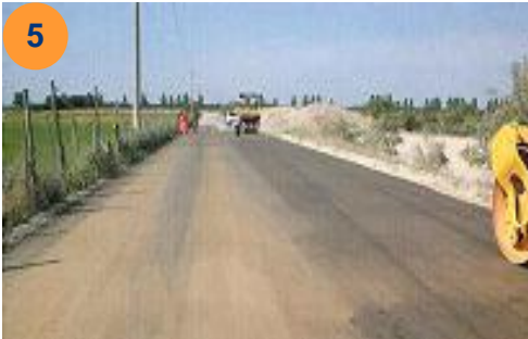
Final compaction
