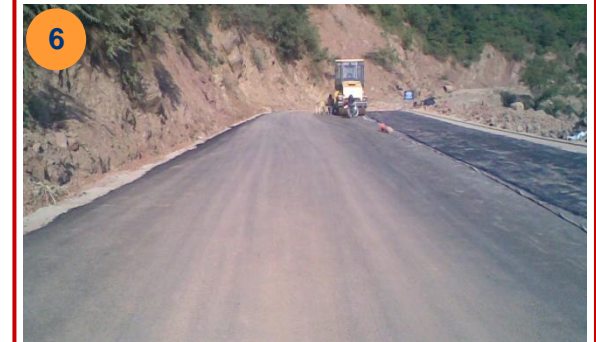
Final road surface
